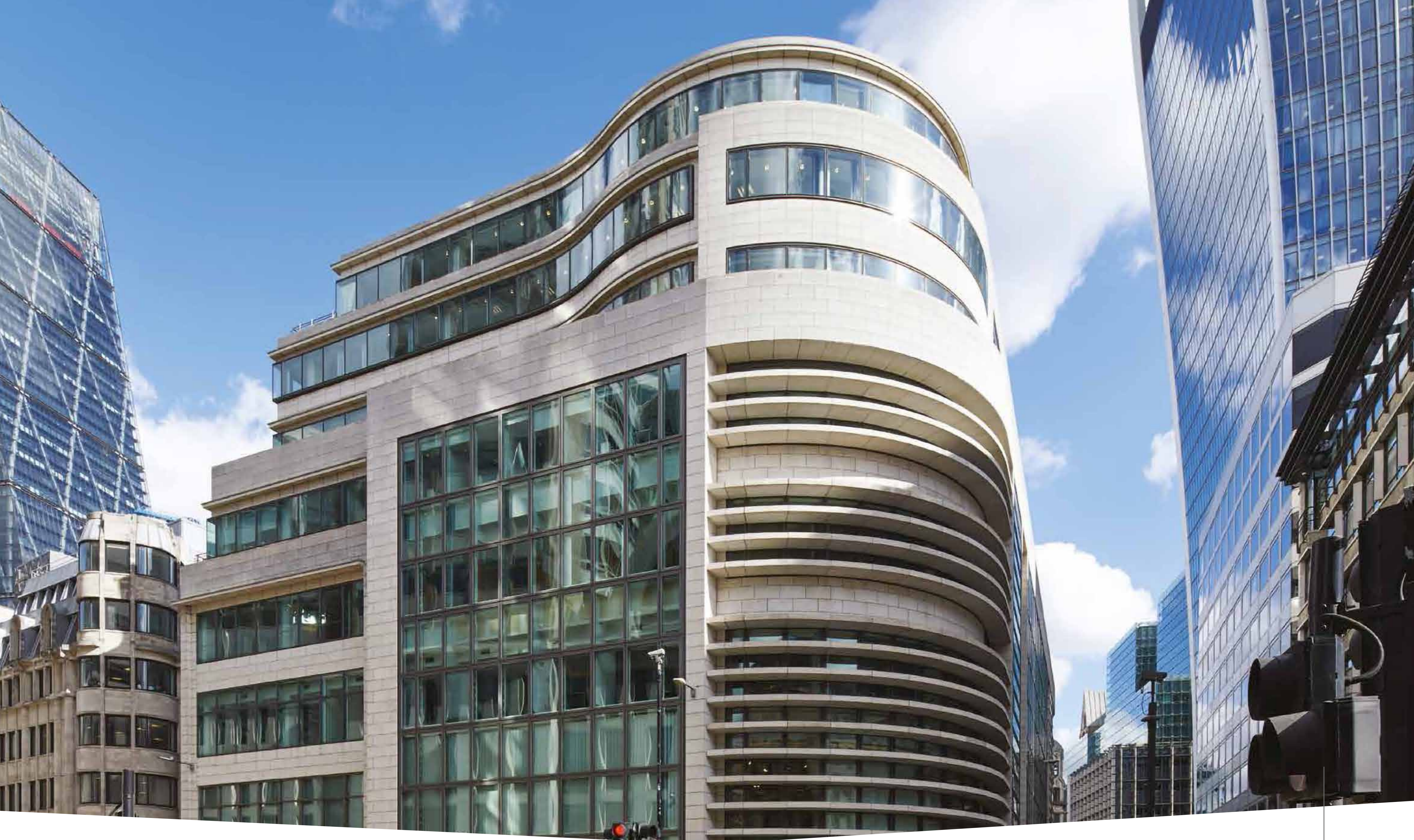
The existing building viewed from Gracechurch Street
