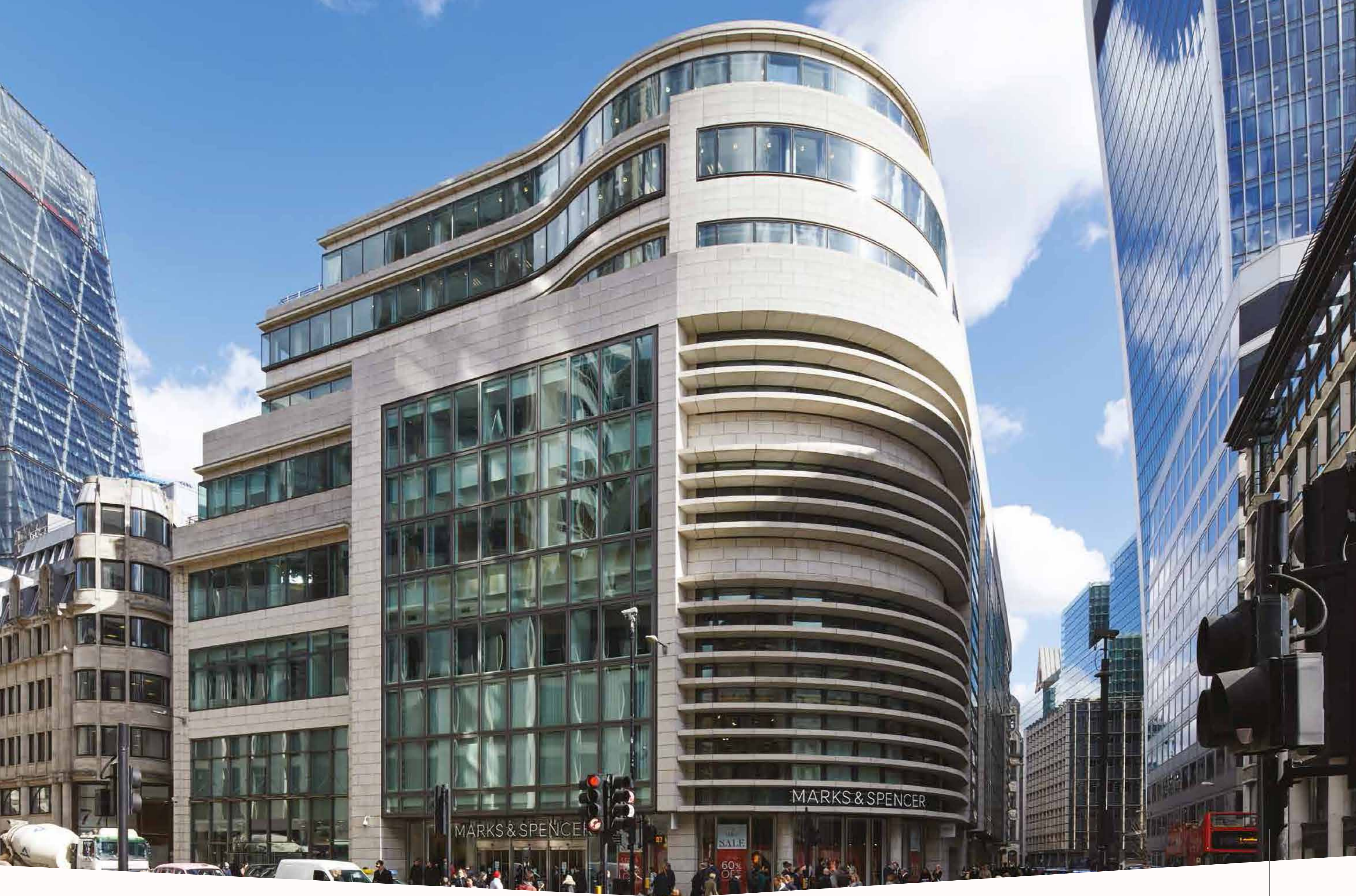
The existing building viewed from Gracechurch Street
